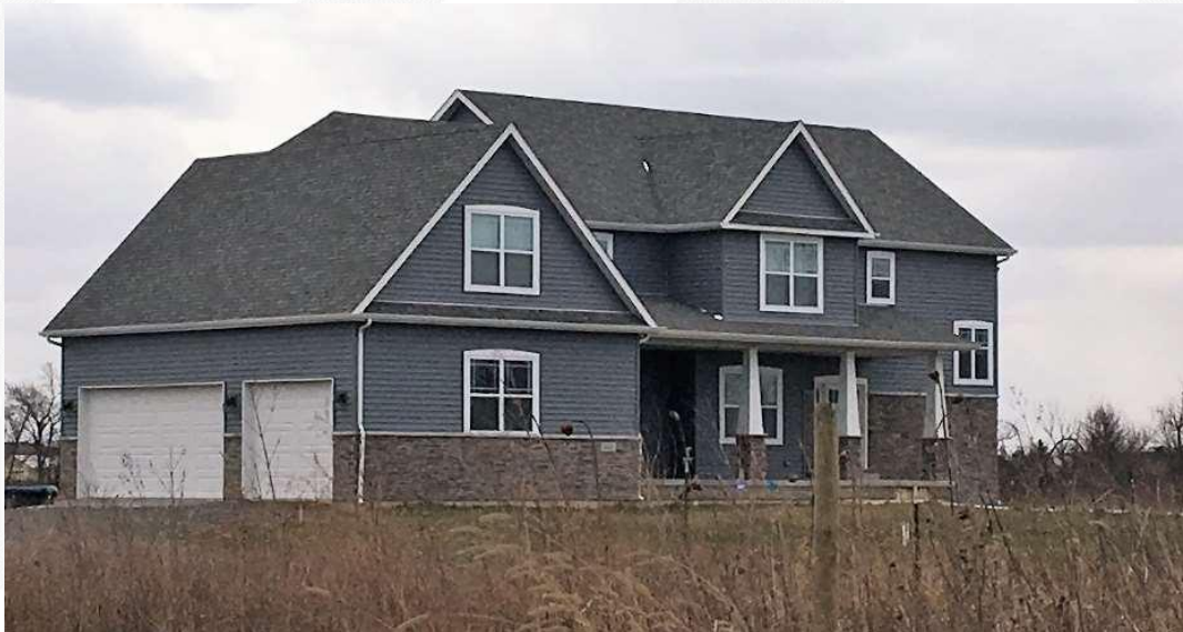
4,255 square foot estate home under construction, adjacent to Portage Solar Farm located in Indiana
