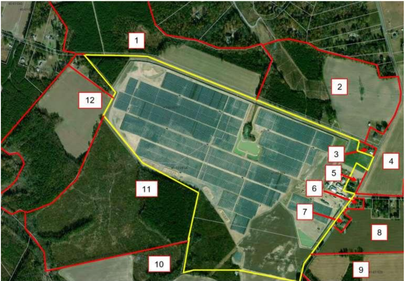
Woodland Solar - Adjoining Properties
